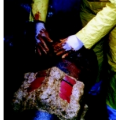
Application of Petrolatum Tape system.
